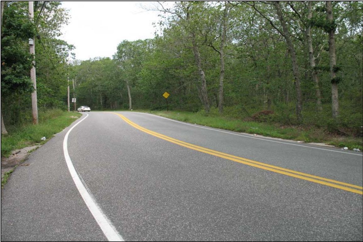
(m): Looking north along Josiah Foster's Path between Montauk Highway and Head of Lots Road.
