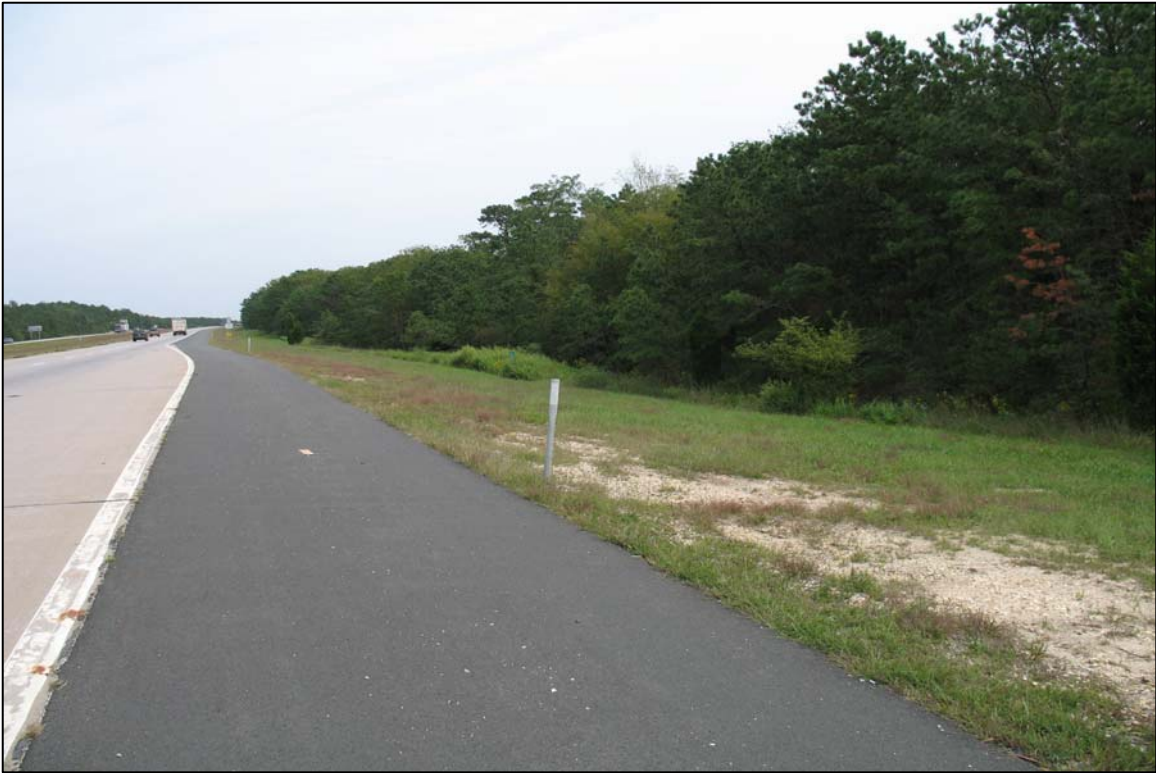
(k): Looking east on Sunrise Highway at intersection with CR 104 toward Central Pine Barrens region on south side of Sunrise Highway.
