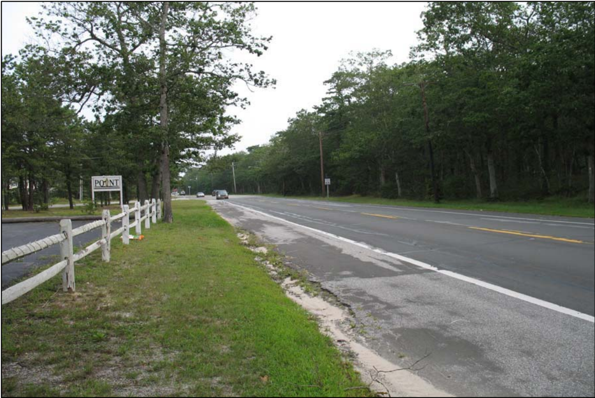
(l): Looking east from Montauk Highway toward intersection with Old Country Road at forested lands on the south side of the roadway. A restaurant is visible on the north side of Montauk Highway in this area.
