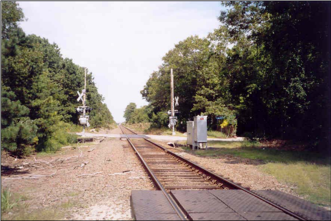
(r): Looking east from grade crossing on Gleason Drive toward grade crossing at Oak Street.
