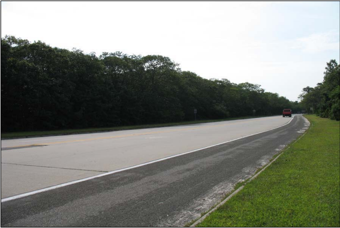
(a): Looking south at Quogue Riverhead Road (CR 104) near Jeffrey Lane.
