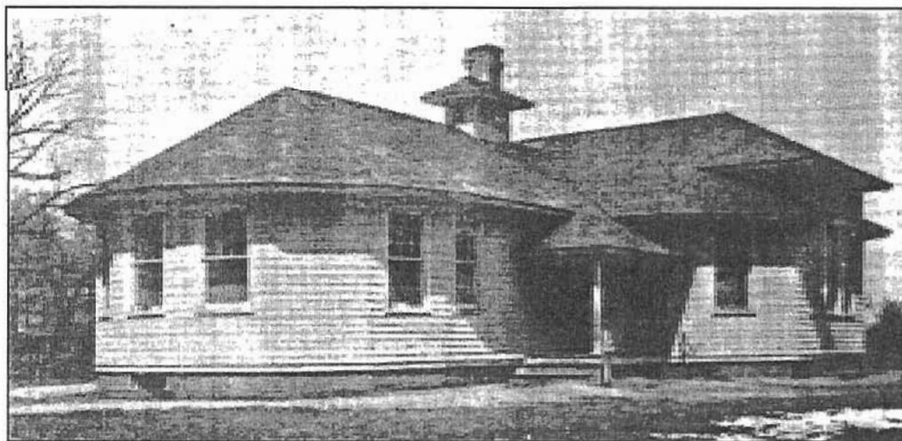
First Eastport School on site
