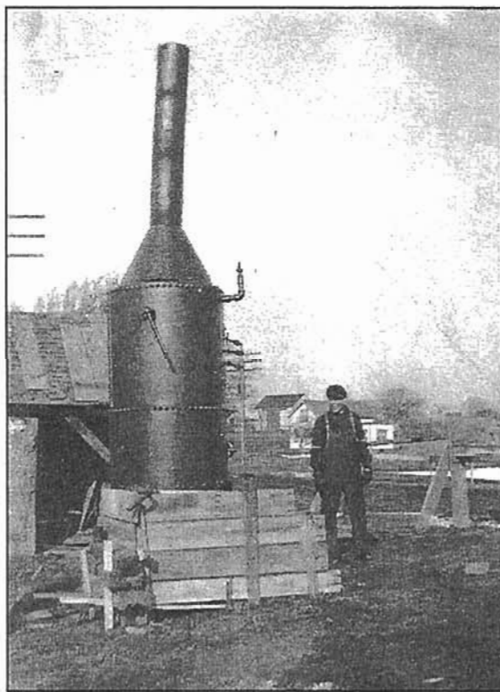
Vertical steam boiler to run saw mill at East Pond
