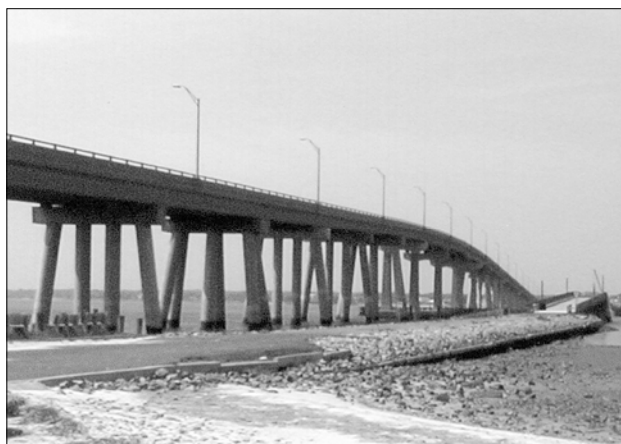
New Ponquogue Bridge Photographed May 2007 Shows remnants of old bridge to the right.
