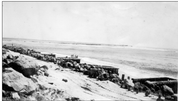
Photograph showing timber cribs filled with stone to stabilize the inlet circa 1940s
