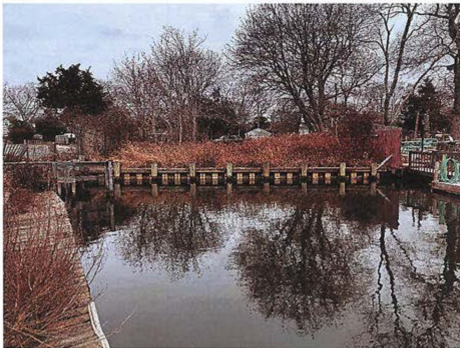
View looking at existing bulkhead. Proposed replacement with low-sill bulkhead.
