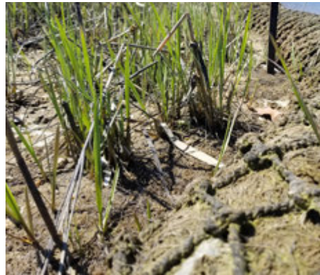
b. Marsh grass will be planted in submerged coir fiber logs/mats within the raft
