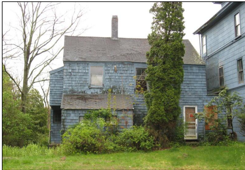
Kitchen addition on the north side of the Brewster House, originally the Flanders Club Headquarters built in 1891. Courtesy of Gary A. Cobb.
