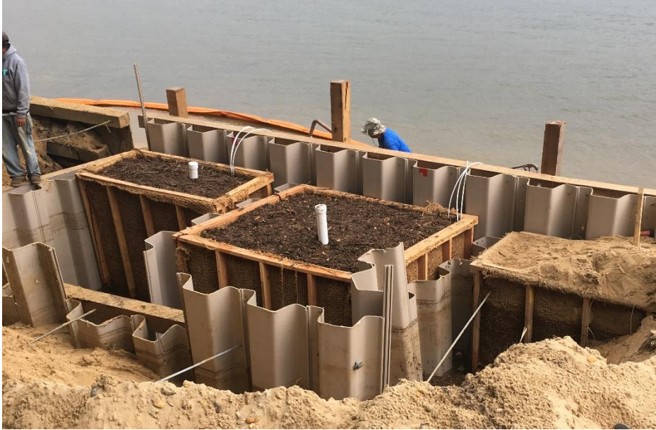
Figure 2. Photo during installation of the bulkhead permeable reactive barrier (PRB) that is trenched into the ground to remove nitrogen in groundwater.
