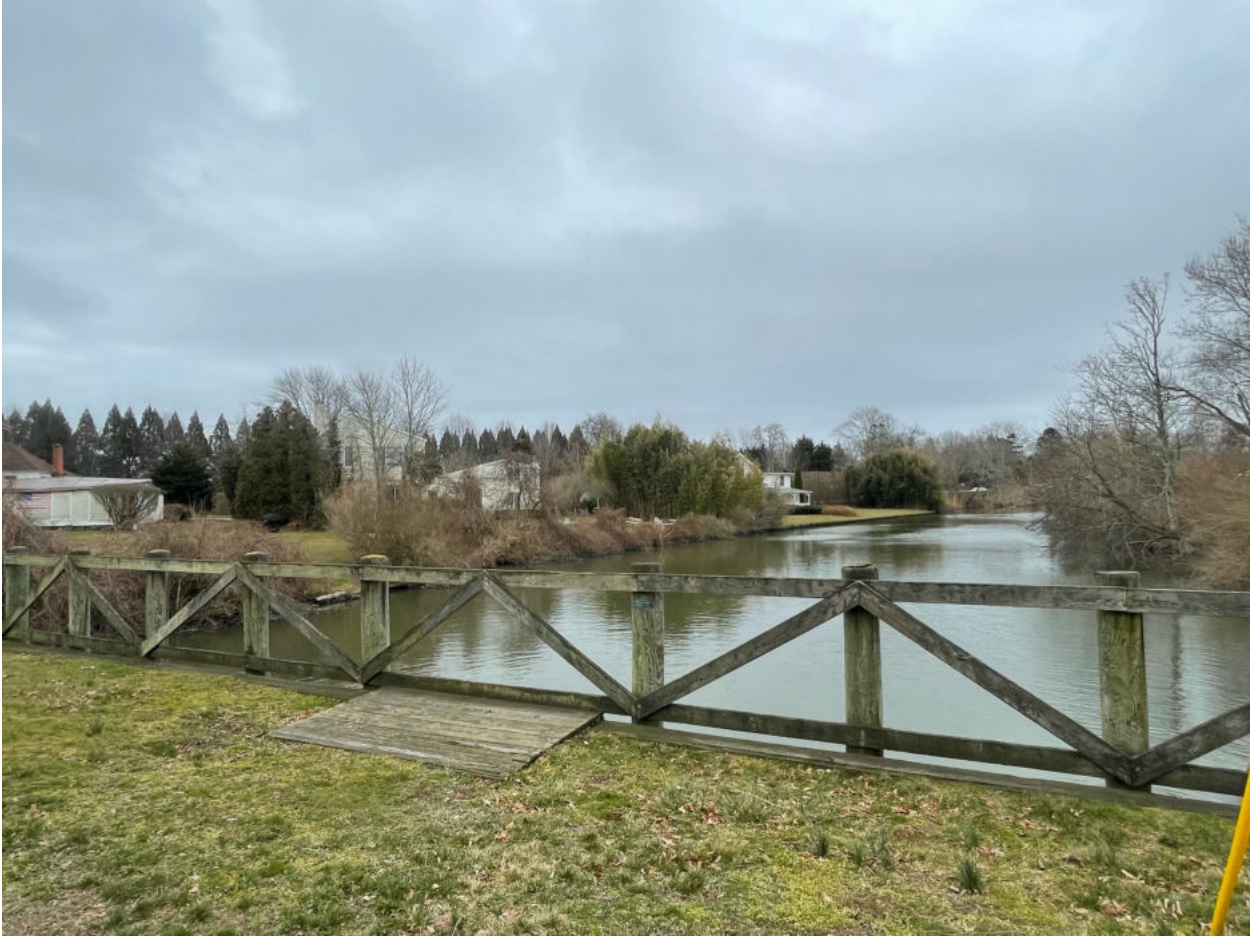
Photo 4. On top of bulkhead, facing South.
