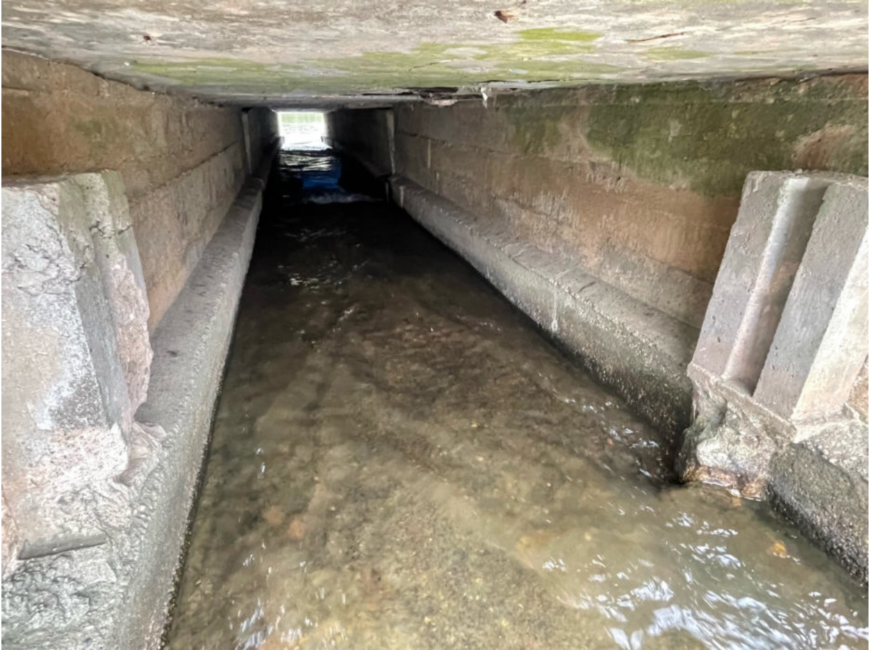
Photo 2. Inside the culvert.
