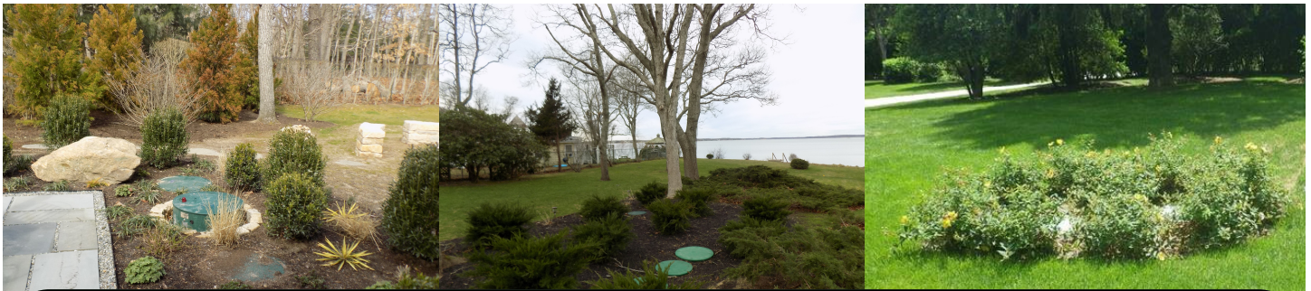
Septic access points are at grade for monitoring and maintenance. Once the system is installed, homeowners can also landscape the surrounding area to enhance the aesthetic appeal.
