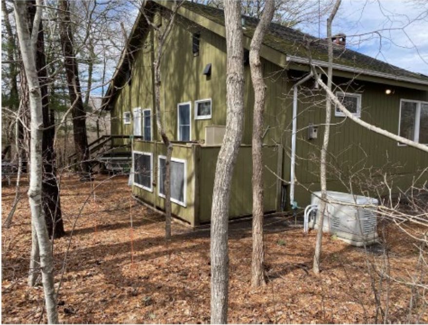
Photograph 3: South side of Nature Center.
