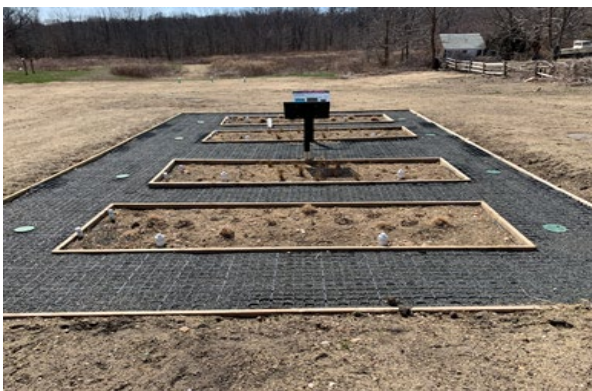
Photo 2 - Vegetated Wetlands Treatment System under Construction
