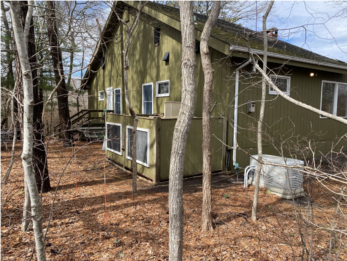
Photograph 3: South side of Nature Center.
