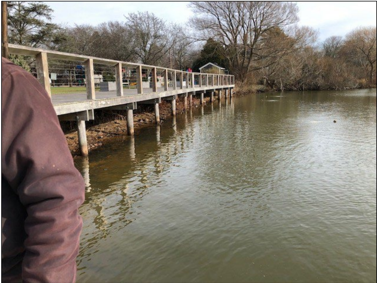
Figure 13: Dock Looking East
