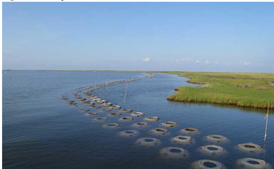
Figure 4: Example of Reef Ball Installation
