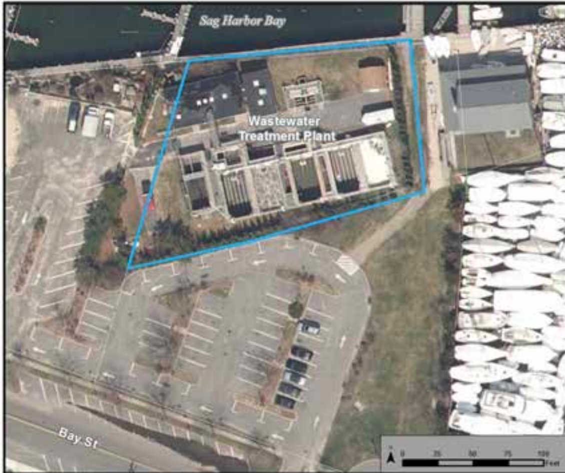
Figure 5. Wastewater Treatment Plant
