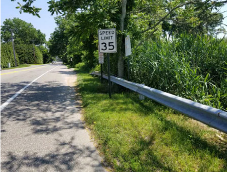
Noyack Road in vicinity of Culvert
