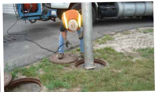
A CDS unit can be easily cleaned in less than 30 minutes
