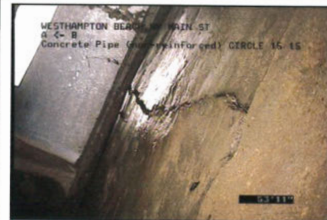
Photo: 6_1_3_13092016_103953_B.JPG, VCR No.: DVD01 TV-91 53.9FT, Upstream Manhole, Survey Ends
