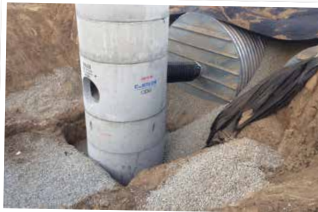
CDS protects detention system from sediment build-up and reduces maintenance
