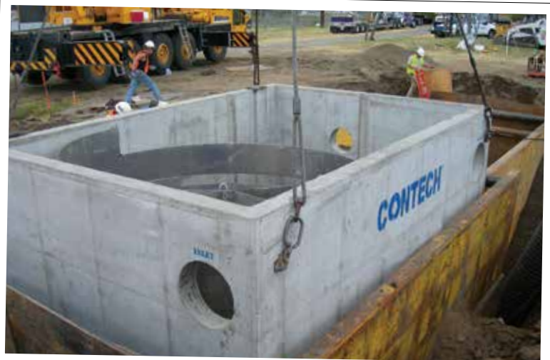
Large diameter swirl chamber for enhancement of sediment removal in a low profile unit
