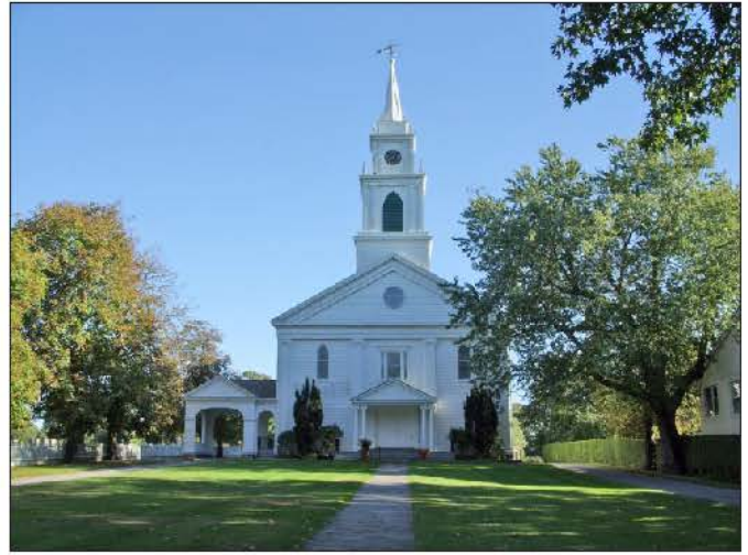
Resource BHHD-104: 104 Previously determined SNR-eligible, the Bridgehampton Presbyterian Church, located at 2429 Montauk Highway, was constructed in 1842. It was designed, most likely by Nathaniel Rogers, in the Greek Revival style. The clapboard-clad building features Ionic pilasters, pointed-arch windows, and the original spire. A port-cochere on the east side, a porch on the north side, and a clock were late 19th century additions
