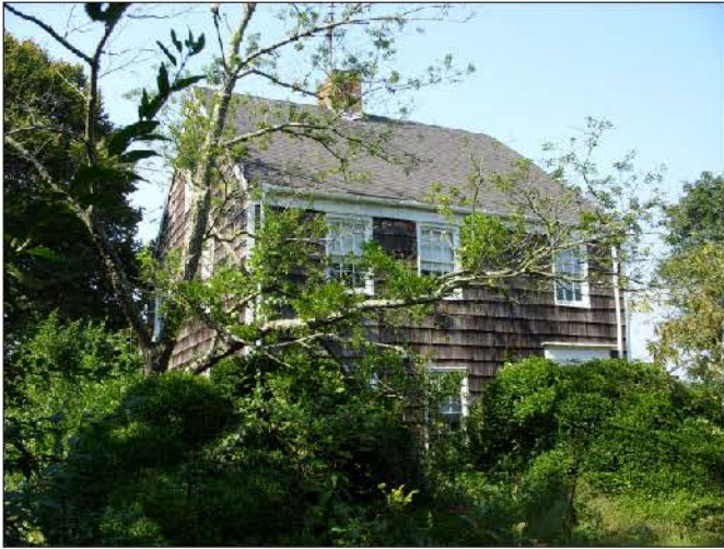
Resource WMHD-16, the David Halsey House, located at 173 15 David's Lane, is an early vernacular two-story three-bay farmhouse with a center chimney, six-over-six-light double-hung-sash windows, and a simple cornice and door surround. Several barns, some of which are in good condition and others in poor condition, are located on the property, as is a potato barn, and a privy. It may be the oldest extant house in Water Mill, built ca. 1750
