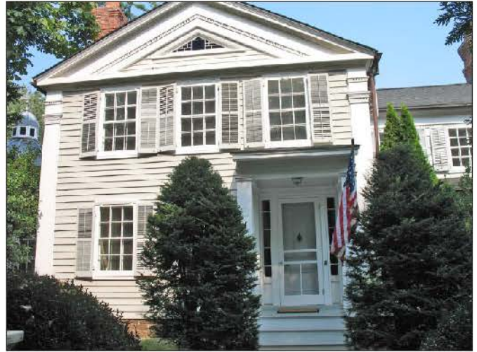
Resource BHHD-68: 68 161 Lumber Lane, the D. Gardiner House, is a three-bay front-gable Greek Revival-style dwelling with a triangular window in the pedimented gable, pilasters, six-over-six-light windows, wood shutters, and sidelights around entryway and original entry porch. The structure has a brick chimney and a brownstone foundation, and was likely constructed ca. 1840
