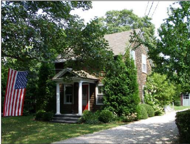
Resource BHHD-37: 37 19 Halsey Street is a one-and-a-half-story three-bay side-gable shingle-clad vernacular dwelling with brick chimney
