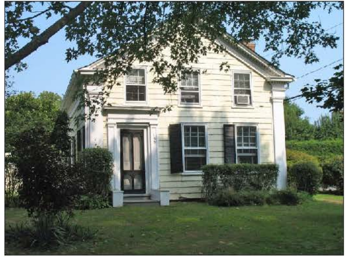
Resource BHHD-66: 66 189 Lumber Lane, the ca. 1840 Jacob Strong House, is a three-bay front-gable Greek Revival-style house, clad in wood clapboard, with pilasters, dentilled eaves, and Greek Revival-style door frame. The house has a brick chimney and six-over-six-light windows
