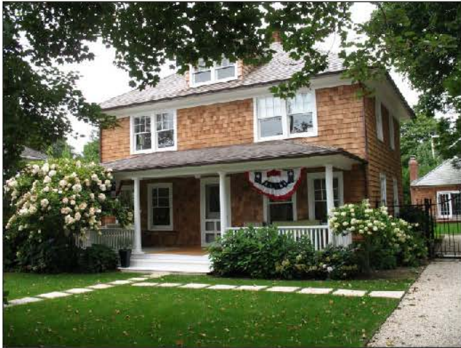
Resource BHH-115: 115 47 School Street is a Prairie-style 'four-square'-form house, clad in wood shingles, with a hip-roofed dormer, hip-roofed porch, and six-over-one-light windows. Like many of its neighbors on School Street, the house was built after the Nathan Hand property was subdivided ca. 1920
