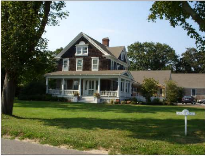
Resource WMHD-18, the ca. 1880 D. Halsey House at 258 Halsey Lane is a two-story cross-gable Queen Anne/Colonial Revival-style dwelling with decorative multi-light windows, and a porch supported by classical columns 17
